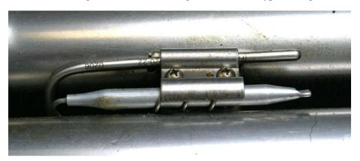
Typical high-limit/sensor probe locations and mounting hardware.
